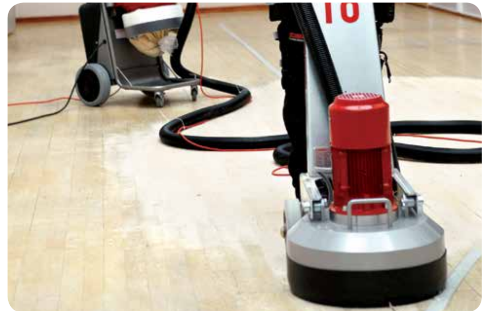
Grinding of hardwood floors and parquet flooring
