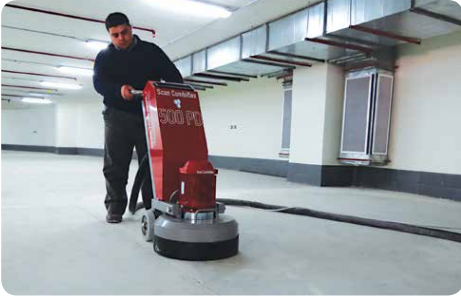
Removal work and floor preparation
